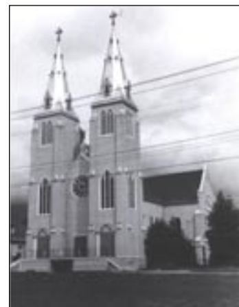
St. Paul's (North Vancouver) was renovated in 1910 during which time a second steeple was added.
